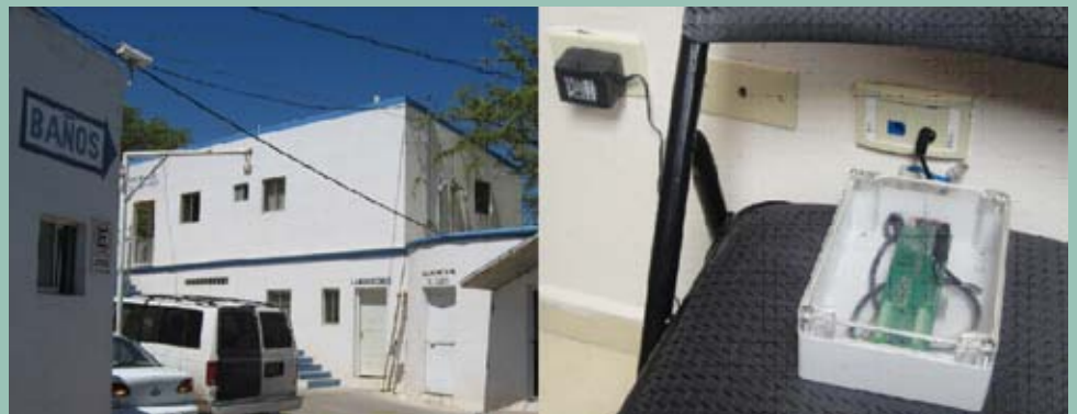
Figure 2. The Nogales, Sonora Water and Wastewater Utility building, site of the first community rain gage in the network (left). Electronic connection that conveys precipitation data from the rain gage directly to the Internet (right).
