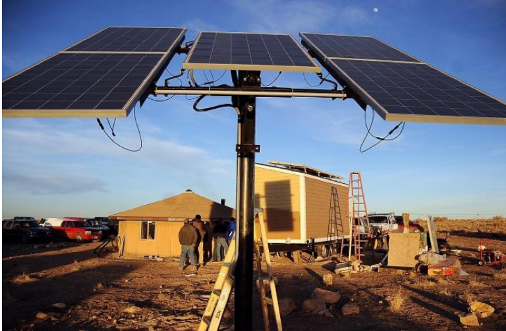
An IINA Solutions residential solar system for an off-grid households (photo credit, IINA Solutions, available at http://iinasolutions.com/ )
