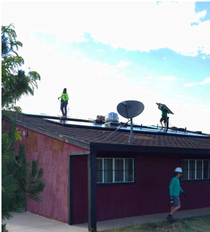
Solar installation in progress (photo by Wahleah Johns)
