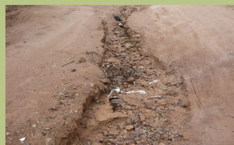
Climate-related vulnerability in a Nogales, Sonora colonia. After heavy rains, unpaved roads in this neighborhood become rutted and uneven.
